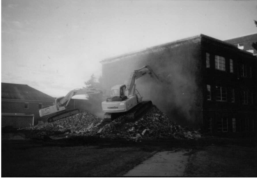
Demolition of Dubs Memorial began on March 29, 2002.
